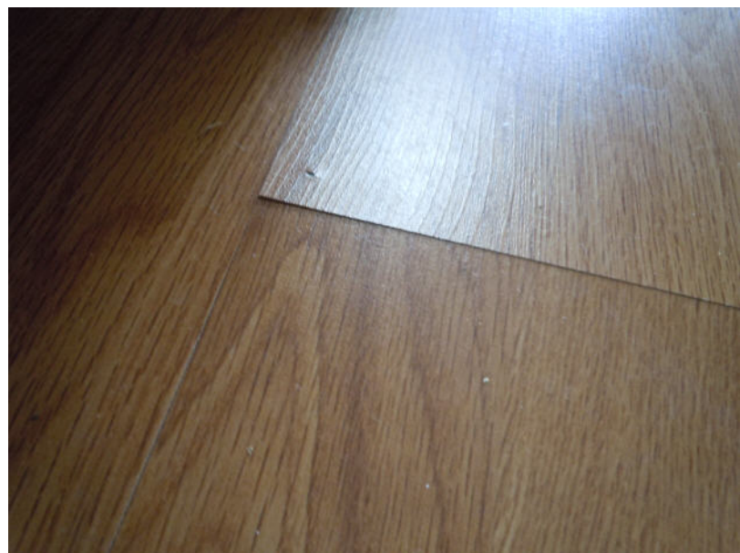
Lifting Laminate, installer nailed down
