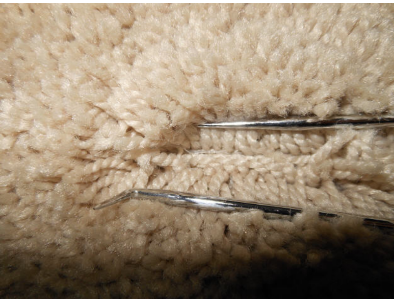
Tufts tucked under seam
