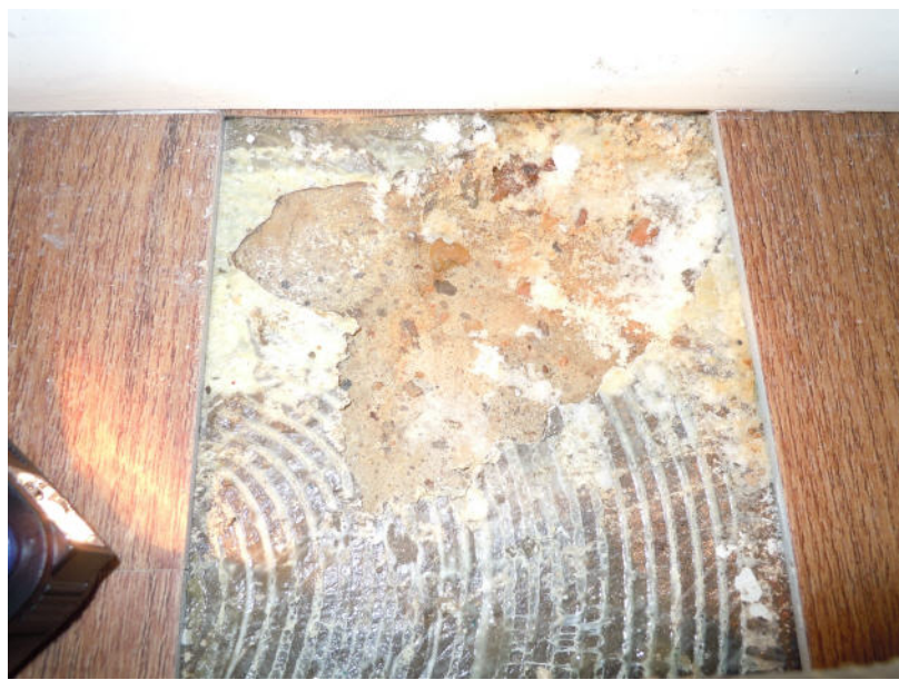
Vinyl planking removed, wet sub-floor with alkali
