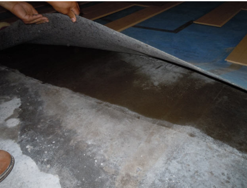
Concrete wet underneath underlayment
