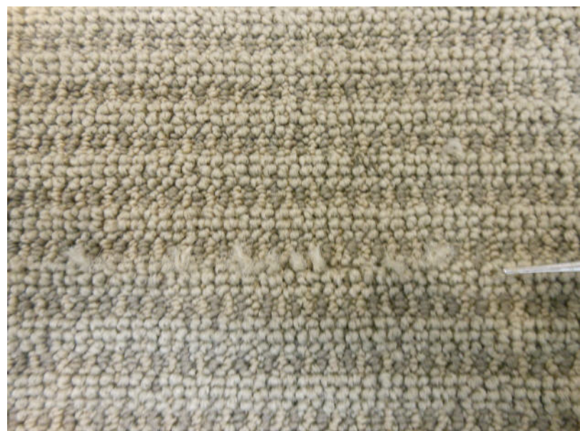
Loops at seam coming apart, no seam sealer
