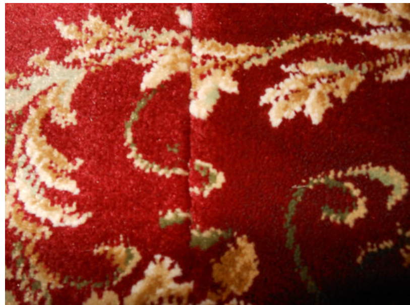
Pattern mismatch and overlapped seam
