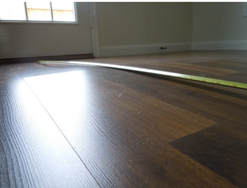
Buckling caused by moisture
