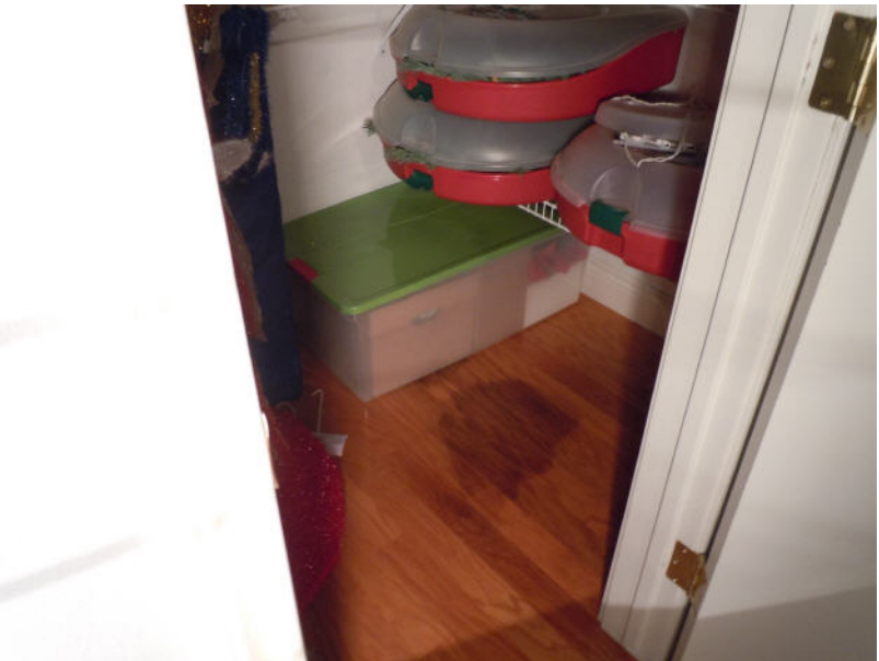
Mold stain coming through to the surface
