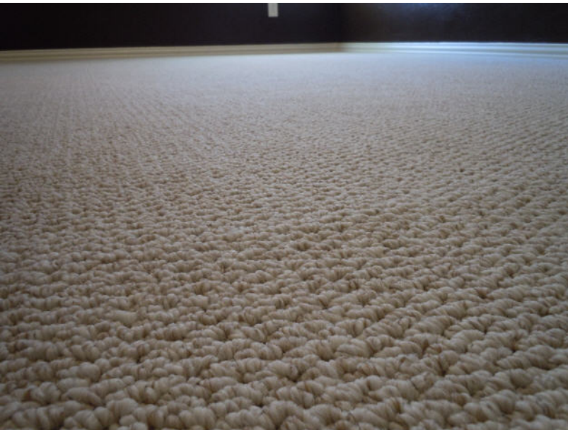
Peaking seam against light source
