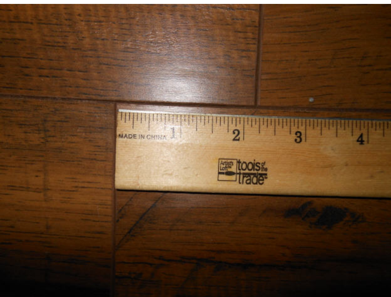
“Out of rack” end joints too close
