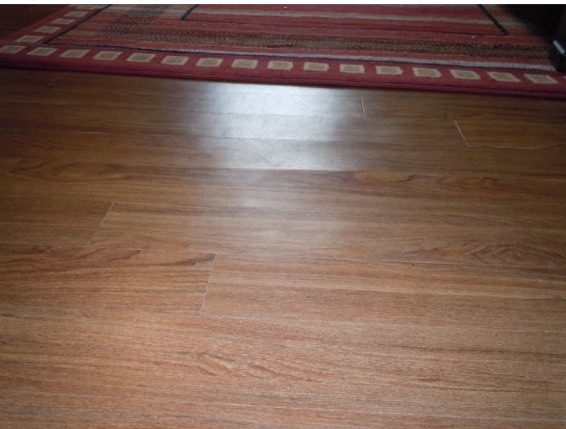
Alkali showing through vinyl planking
