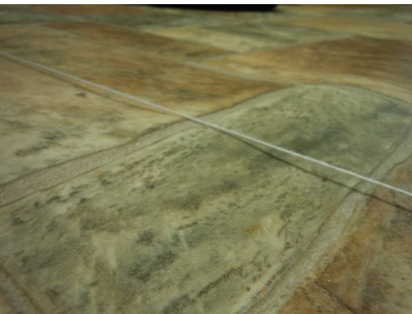
IVC with bubble in center of room
