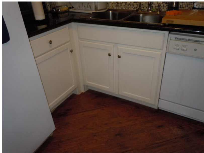
Kitchen counter with granite installed on top of Laminate
