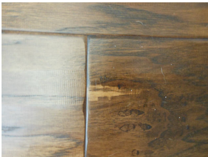
Void in stain underneath surface
