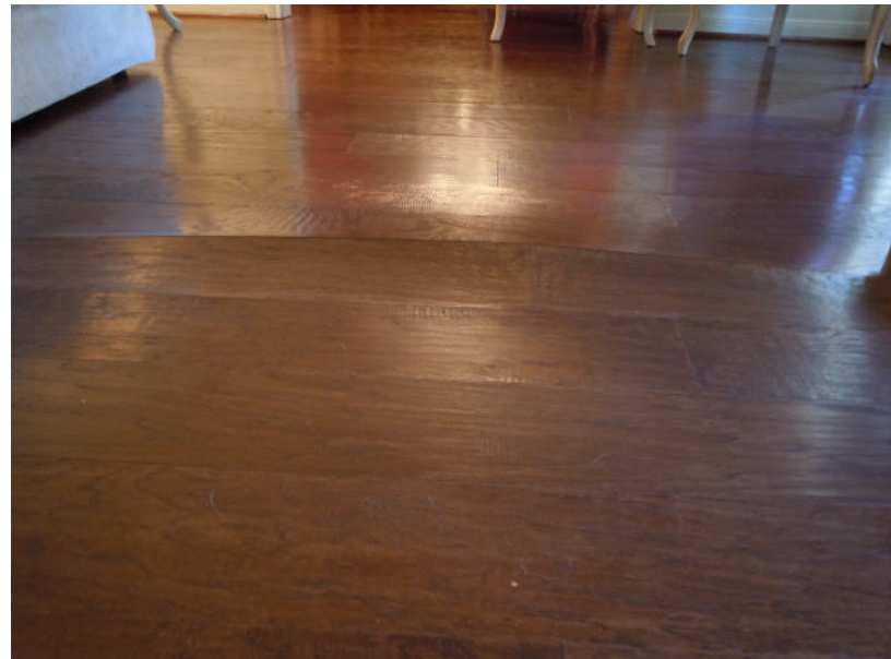
Buckle caused by moisture
